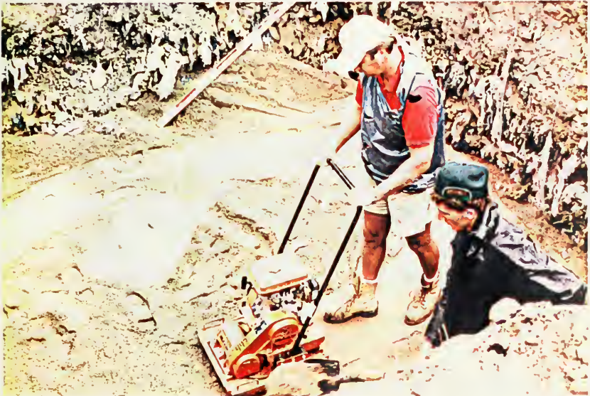
A4: PREPARING BASE
